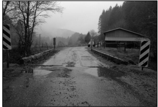
Bridge approach work is a typical ongoing maintenance need for western Oregon roadways. Ditch clearing needs and culvert replacements are also in constant demand.
