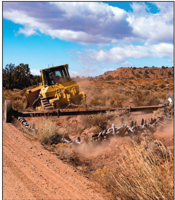
A sagebrush treatment by Dixie harrow in Grand Staircase-Escalante National Monument. (Photo: Ray Bloxham)
