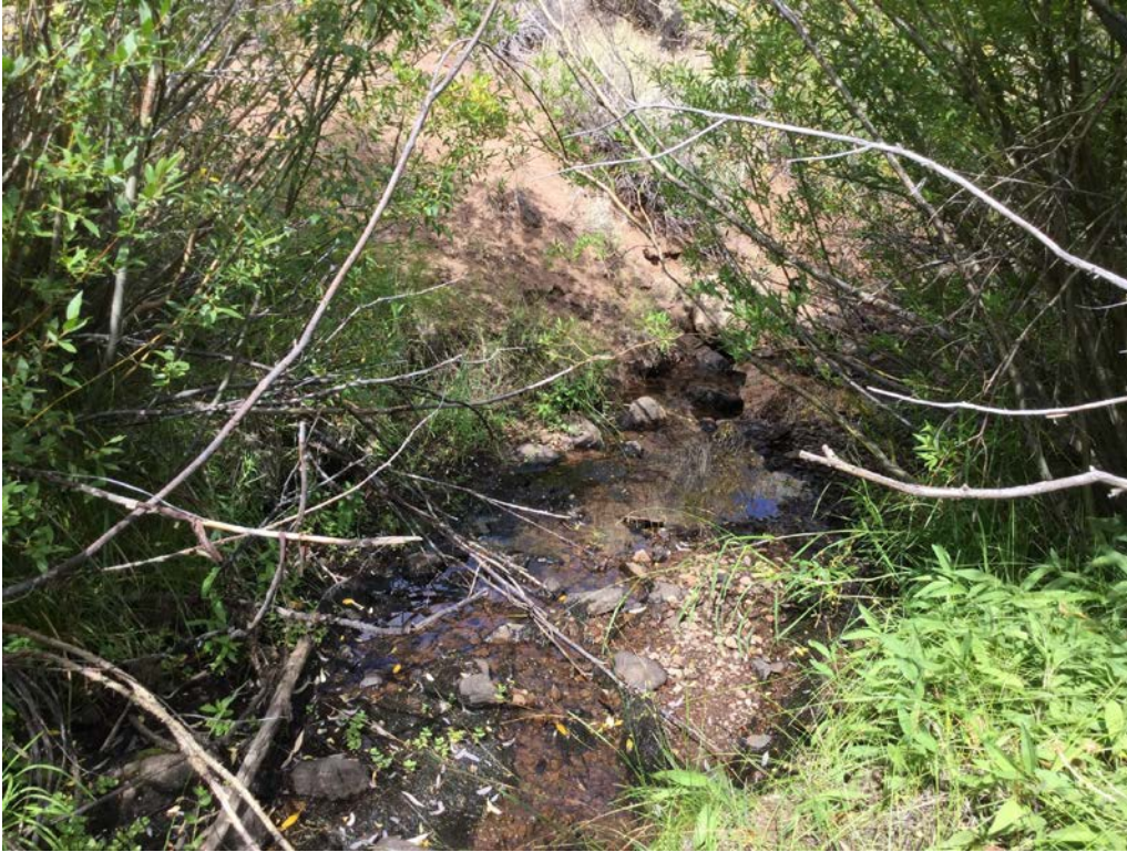
Figure 25 Cabin Pasture, Big Fir Creek DMA, upstream view September 4, 2019
